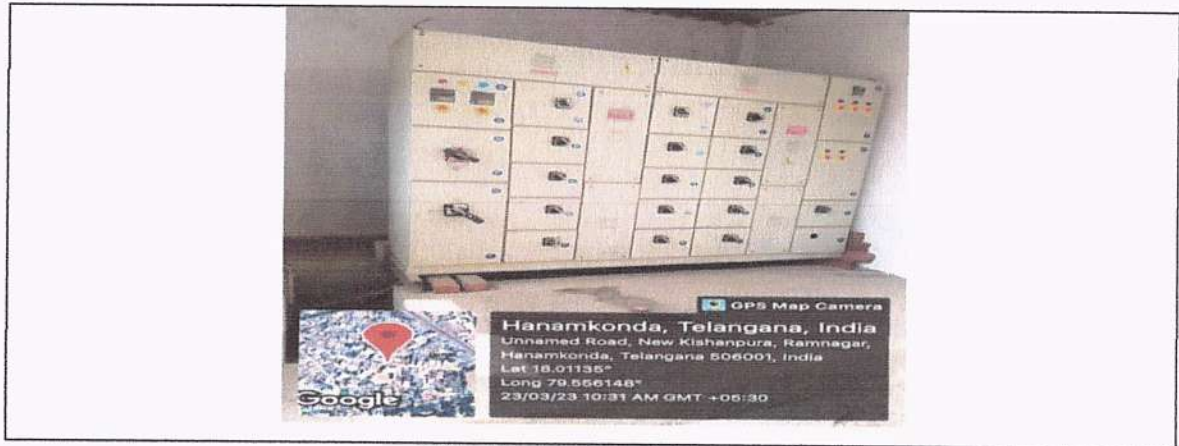
Wheeling to the Grid
