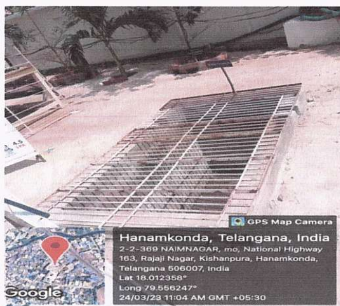
Water Harvesting Pit
