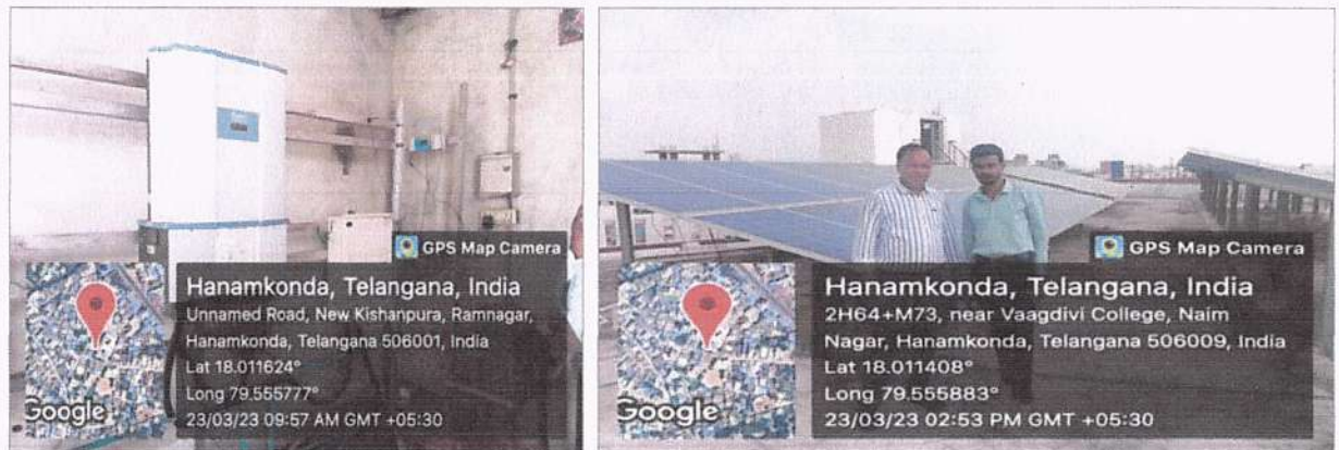
Investigative parameters – Energy Management – Solar panels and electrical appliances
