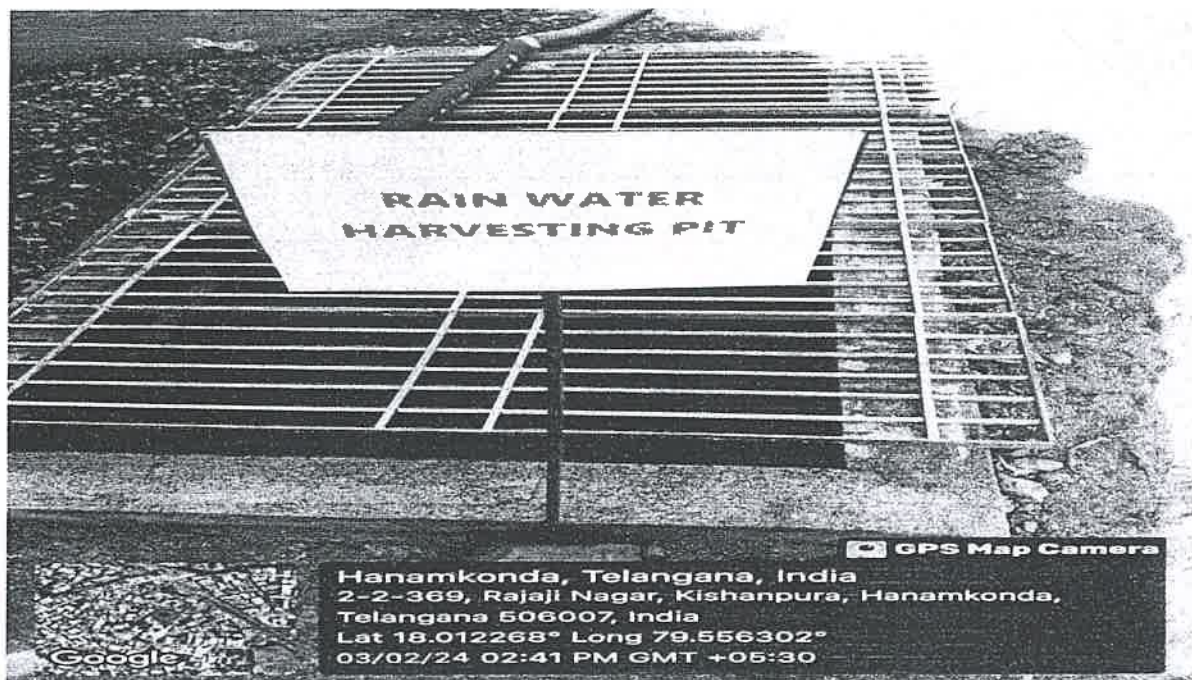
Rain Water Harvesting Pit
